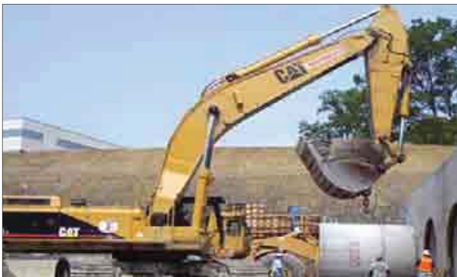
Excavator in action
